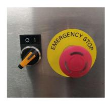
Rotate the eletrical switch to position 0
