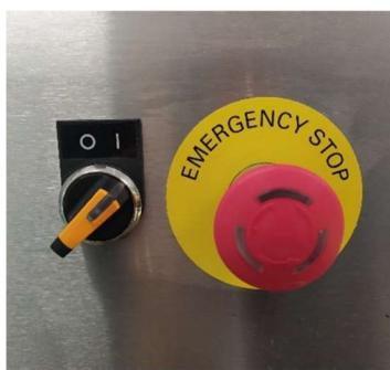
Rotate the electrical switch to position 0
