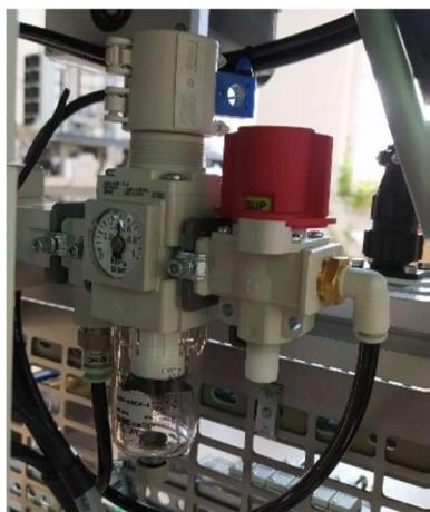
Rotate the station air switch to position sup
